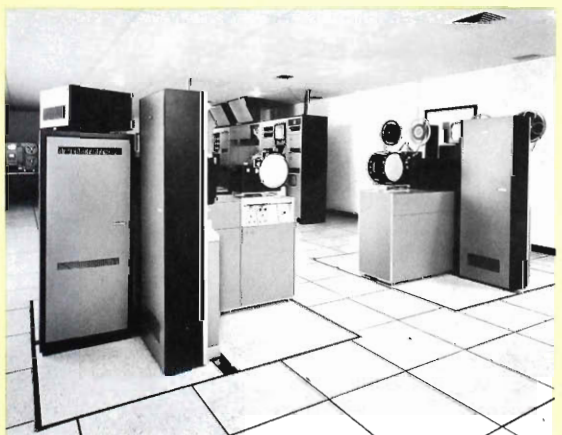
Two conveniently positioned TK-27 film islands handle TV-26 film requirements. Floor space is available for additional film systems when needed.
