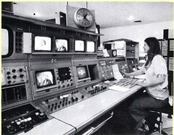
Straight-line control console is laid out with audio and on-air video switching positions at one end; TK-44 camera control units at opposite end.
