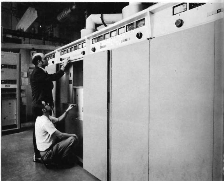
TTU-60, 60 kW transmitter for TV-26 is centrally located on the 50th floor of One Shell Plaza.
