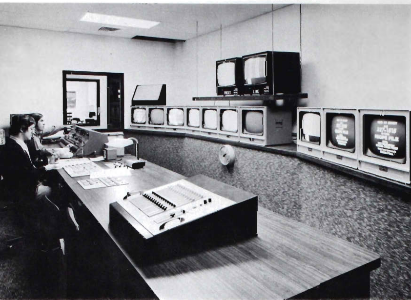
Production control room displays outputs from live, tape and film sources for convenience of director. Remote dimmer control board is in foreground.
