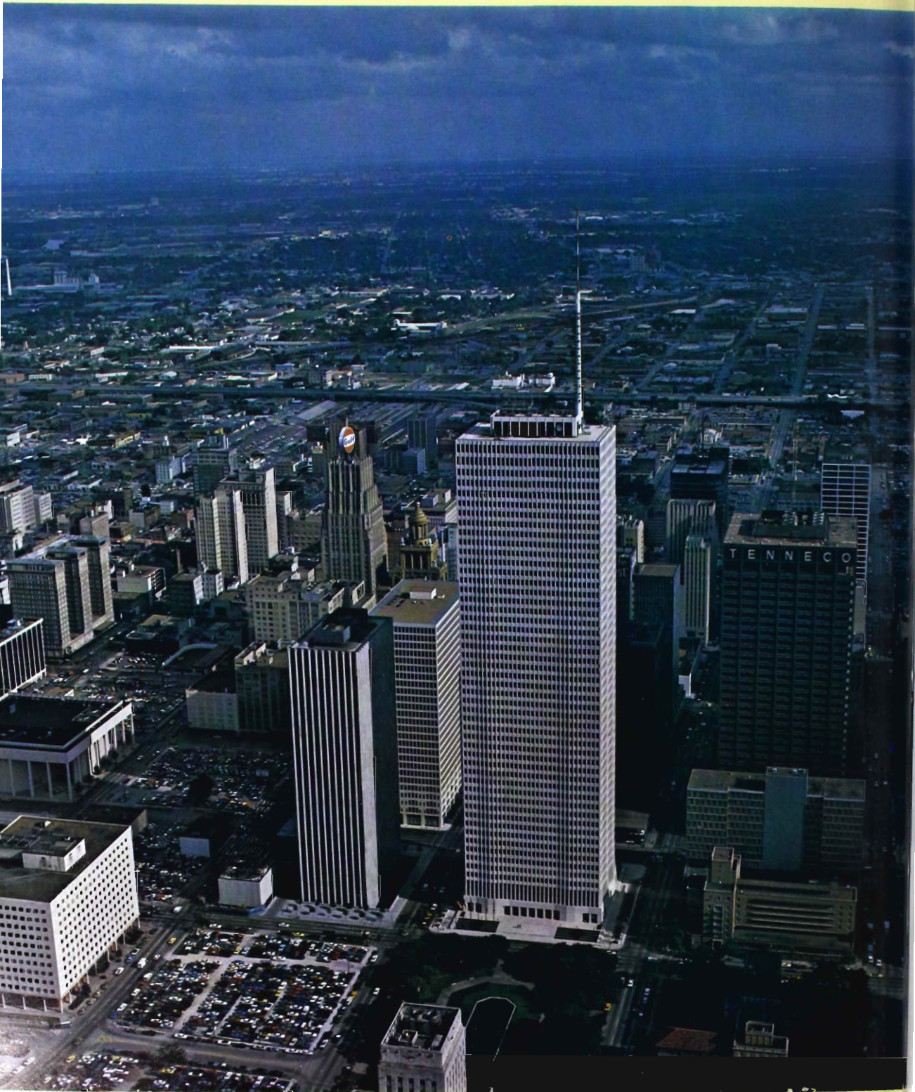
KVRL's omnidirectional antenna atop One Shell Plaza in downtown Houston covers the city with a clear, unobstructed TV signal.
